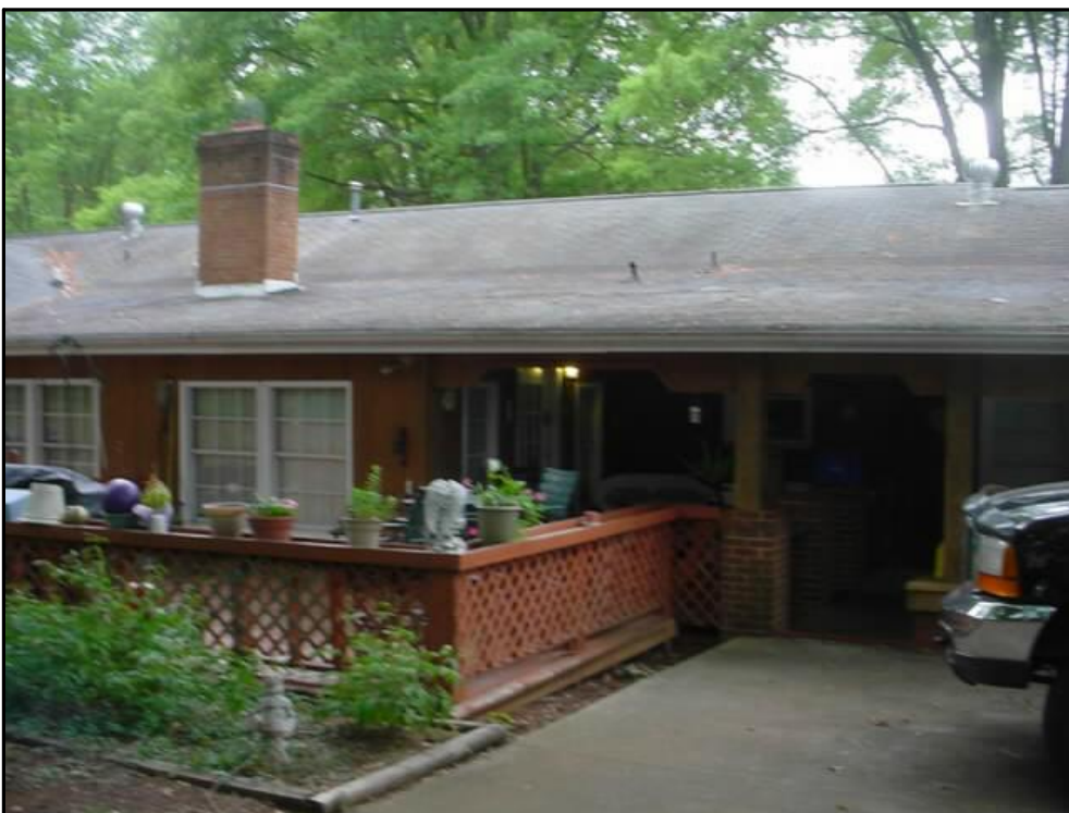
510 DALLAS STREET GENERAL VIEW 6
